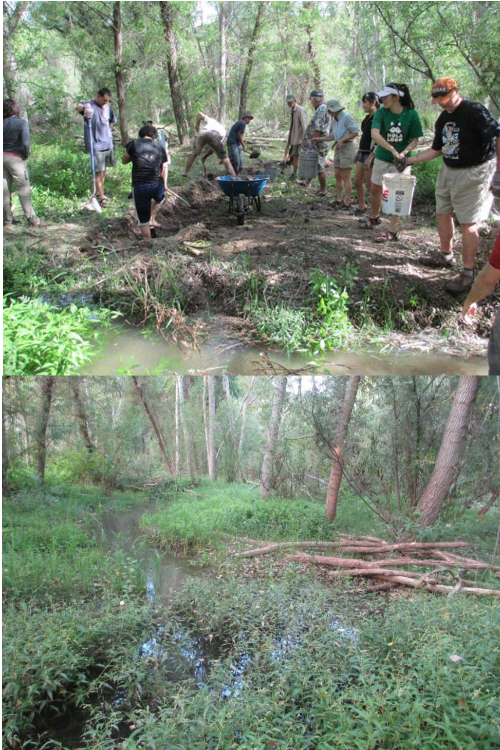
Figure 2: Three Plug & Pond structures installed at Rancho El Aribabi (Robles) to reconnect spring water to historic channels from which it had been cut off. Top: before, May 2013 (dark tree above wheelbarrow is reference point). Bottom: after, August 2013 soil from old channels and logs were used to build earthen dam diversions and protect dams. Water now flows to the Río Cocóspera via surface and subsurface flows from the source of the ciénega.
